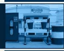
HDG Tanks fire system have been provided with the latest firefighting equipment, which fills the tank from top to bottom with water and foam to suppress the fire. Additionally, there is a separate water tank which has been connected to all tanks in the storage facility. We inspect the tank daily to ensure it is full and ready to be used for firefighting purposes when needed in conjunction with or fire suppression system.
